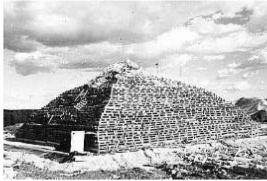
Figure 1: Leachate evaporation pyramid at Hogbytorp landfill, Sweden
